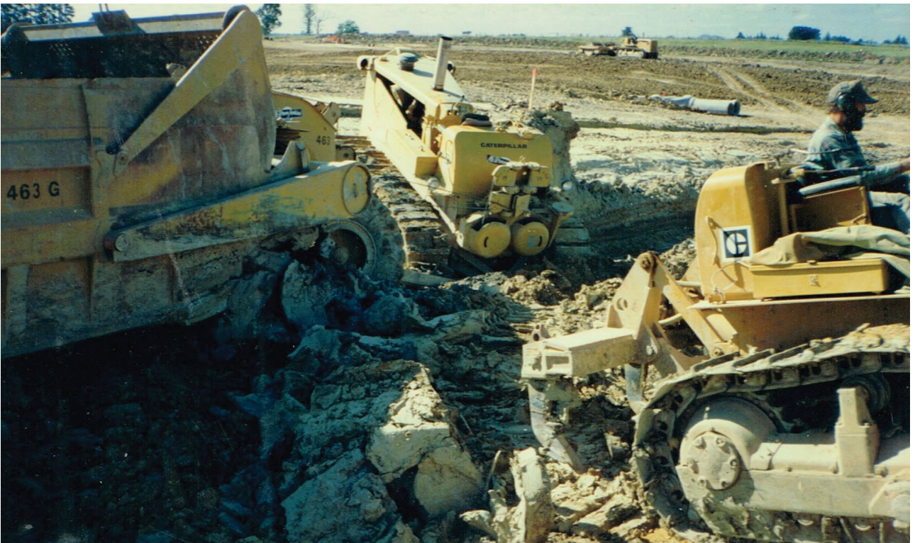
Contouring land for a subdivision: HEB company files
